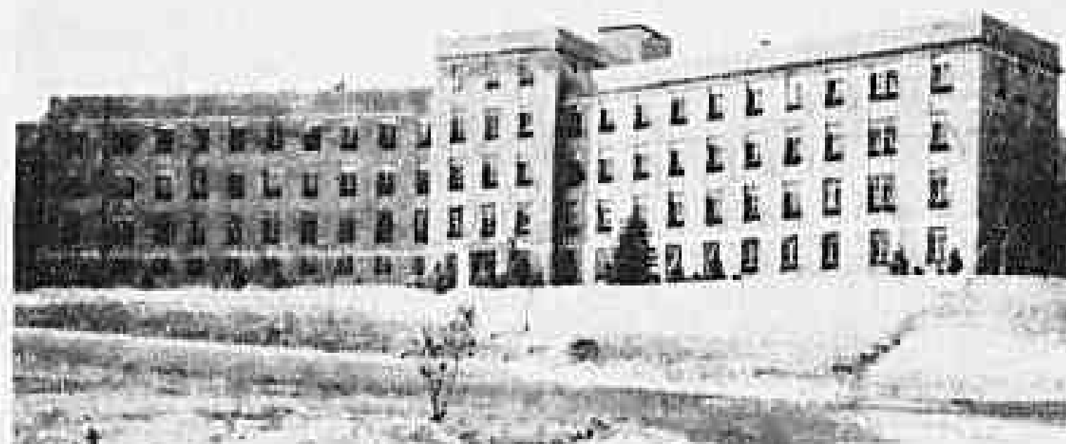
The Mt. Washington Sanitarium, Fairbairn, Wisconsin, Equipped with the new Ceco Intermediate Casement.
